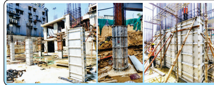
Column Formwork
